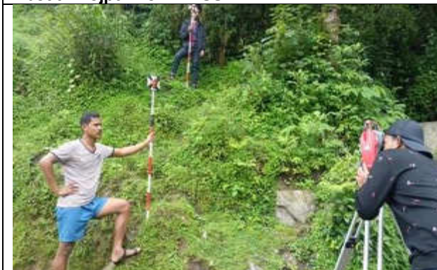
Photo 12: Engineer Is Surveying Transmission Pipe Line By Total Station
