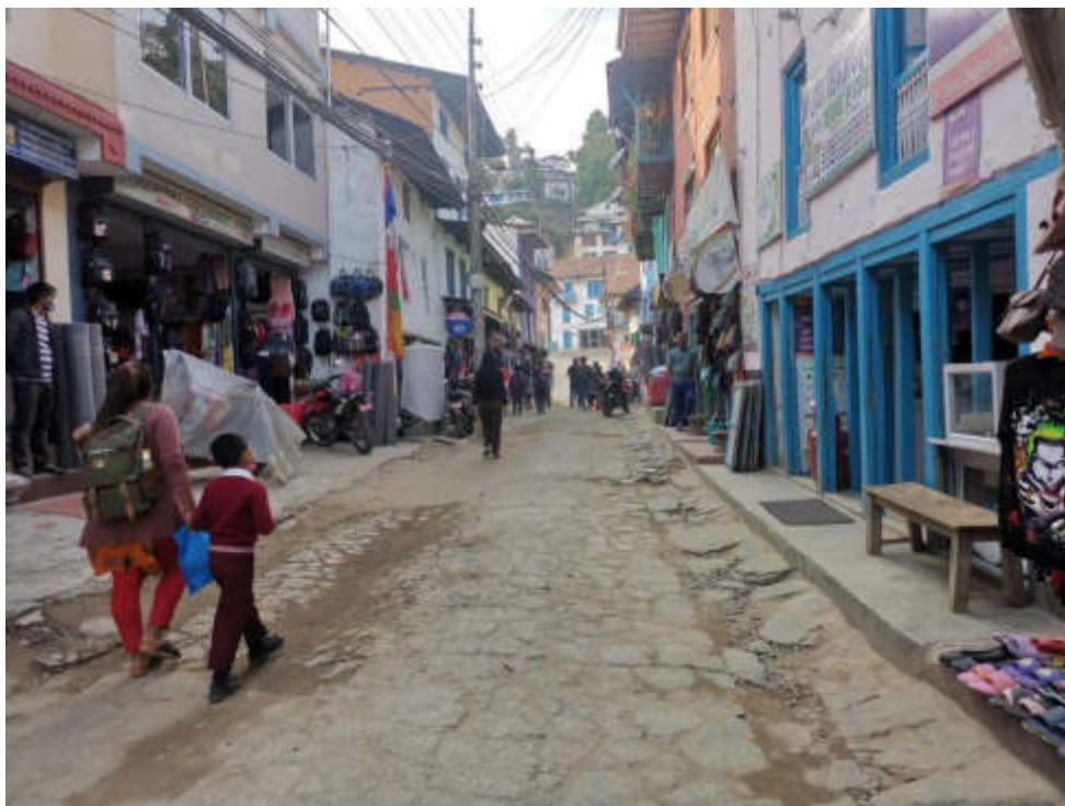
Bhojpur Bazaar Area where sewer pipe is proposed to be laid
