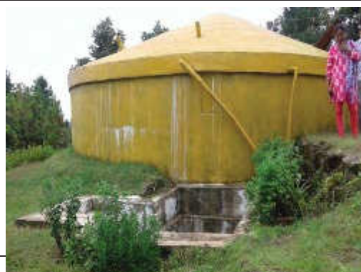
2. Existing RVT at Pani Tanki Area
