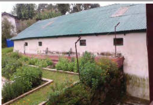
3. Existing RVT at Pani Tanki Area
