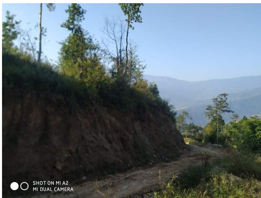
Existing road to WWTP-1 site, Ramkot (Gairawari), ward no 6
