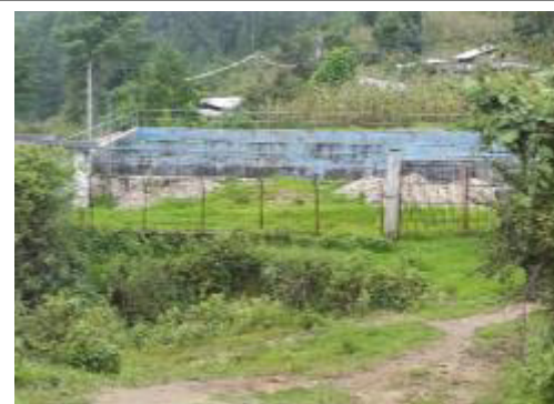
10. Existing WTP (WTP-E)
