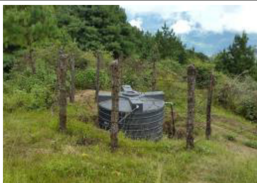
13. Existing WS Scheme near Tower
