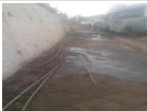
9. Existing Condition of Distribution Pipelines
