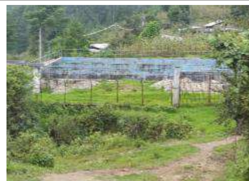
10. Existing WTP (WTP-E)
