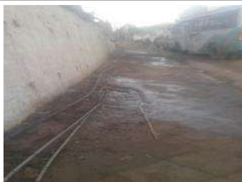
9. Existing Condition of Distribution Pipelines
