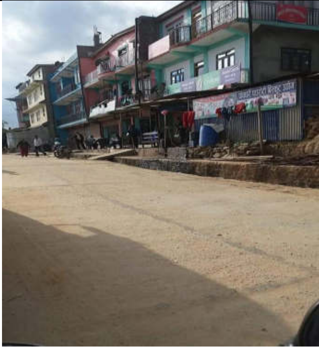
Main Bazar area, sufficient width/ROW for transmission and distribution pipelaying
