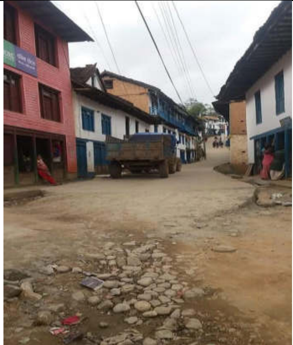
Main Bazar, distribution pipelaying on the way to District Coordination Committee office
