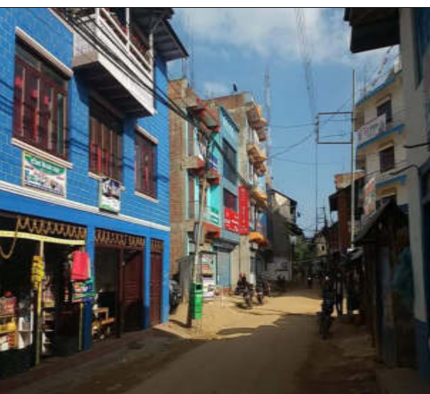
Bazer area, ROW for distribution pipelying
