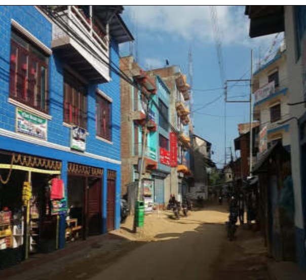
Bazer area, ROW for distribution pipelying
