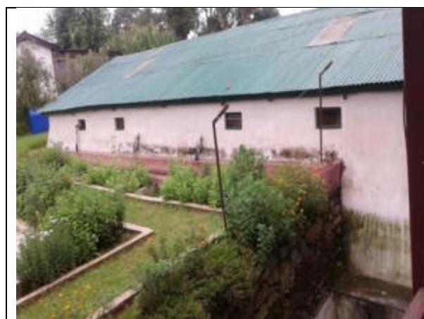
Existing RVT (200cum) at Pani Tanki Area
