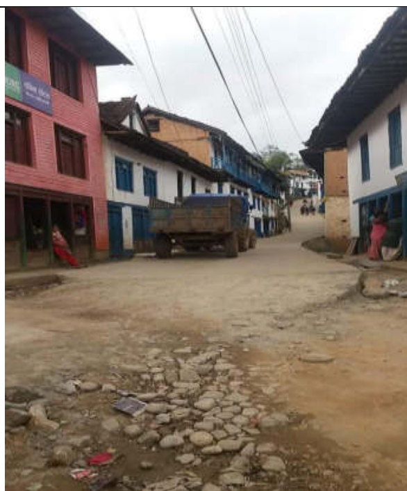
Main Bazar, distribution pipelaying on the way to District Coordination Committee office
