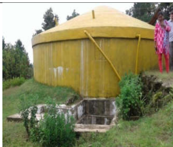
Existing RVT (150cum) at Pani Tanki Area
