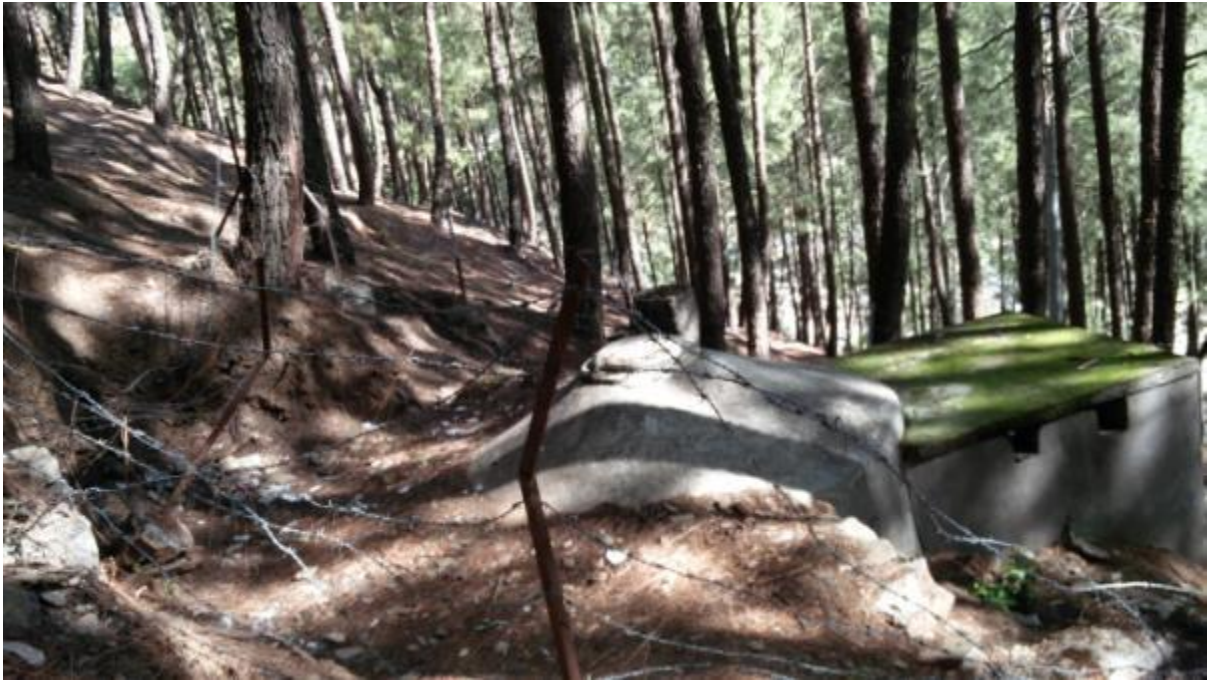
Existing RVT for Bhopur Supply System. The same site will be used for proposed 60 Cum RVT for Bhopur system as shown in photograph below
