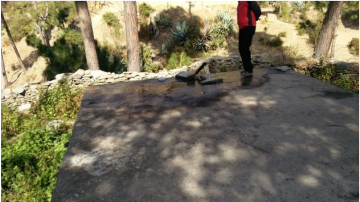
Existing RVT for Water Supply to Chainpur Bazar. The land is already owned by WUSC and same site will be used for proposed 450 RVT as shown in photograph below
