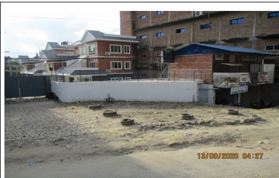
Photo 2: Proposed deep boring site near Dakshin Barahi temple at Dakshinbarahi, Ward No. 4
