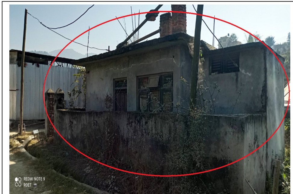
Photo 8: Proposed deep boring, WTP and Guard house site at Sikaritar, Ward No. 4 (Dismantling units shown in red circle).
