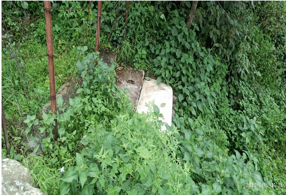
Photo 18: Proposed spring intake site at existing spring intake, Syangtang - Ward No. 4
