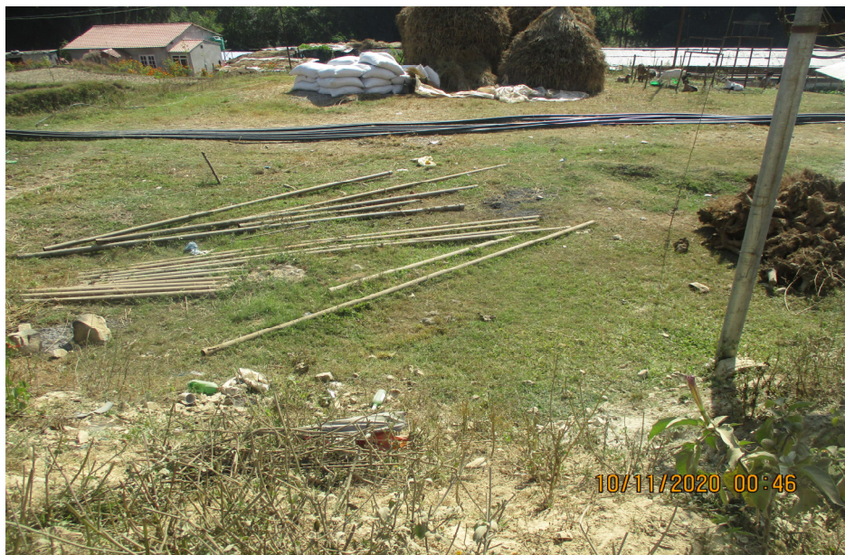
Photo 6: Proposed OHT site at existing ground reservoir tank at Charkhandi, Ward No. 4
