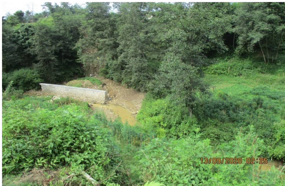
Photo 12: Proposed deep boring site at Ward No. 1
