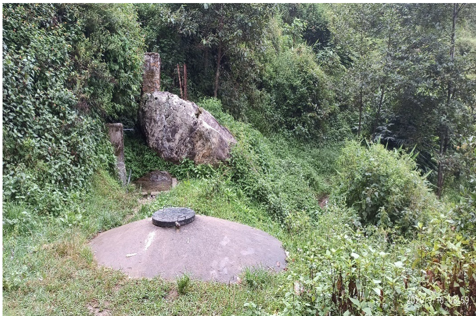
Photo 19: Proposed GRVT site at existing tank, Syangtang - Ward No. 4
