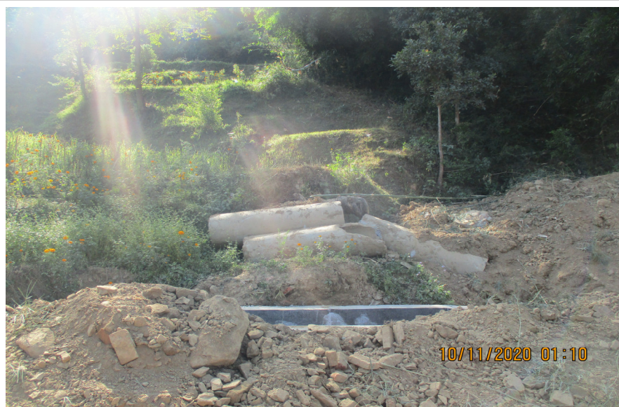
Photo 15: Proposed deep boring site at Birkhaman ko pasal mathi, Ward No. 4. Contractor will relocate abandoned Hume pipes in vacant place with consent from WUSC and local authority
