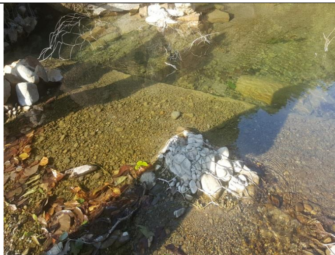
Proposed/ Existing Intake, Pathar Khola, ward no.4
