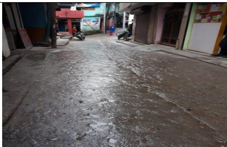
Right of Way where distribution pipes will be laid
