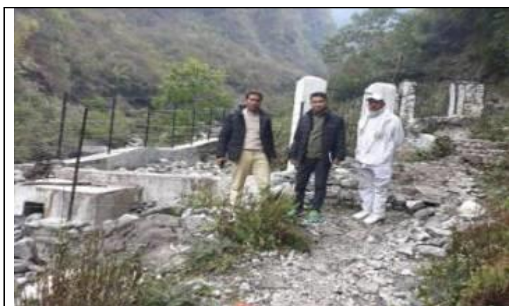
Existing Intake site at Garaku Mul-1 and Mul-2 located at ward no. 3,
