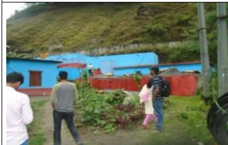
Existing Bangabagar System ward no. 4
