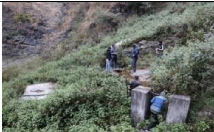
Existing Structure of Galphai System ward no. 5
