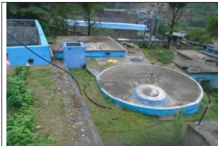
Existing Bangabagar System ward no. 4
