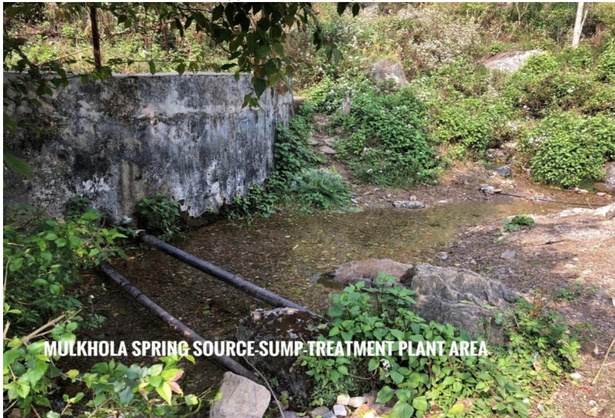
1. Proposed Mulkhola Source for Sump Well, Intake, and WTP.
