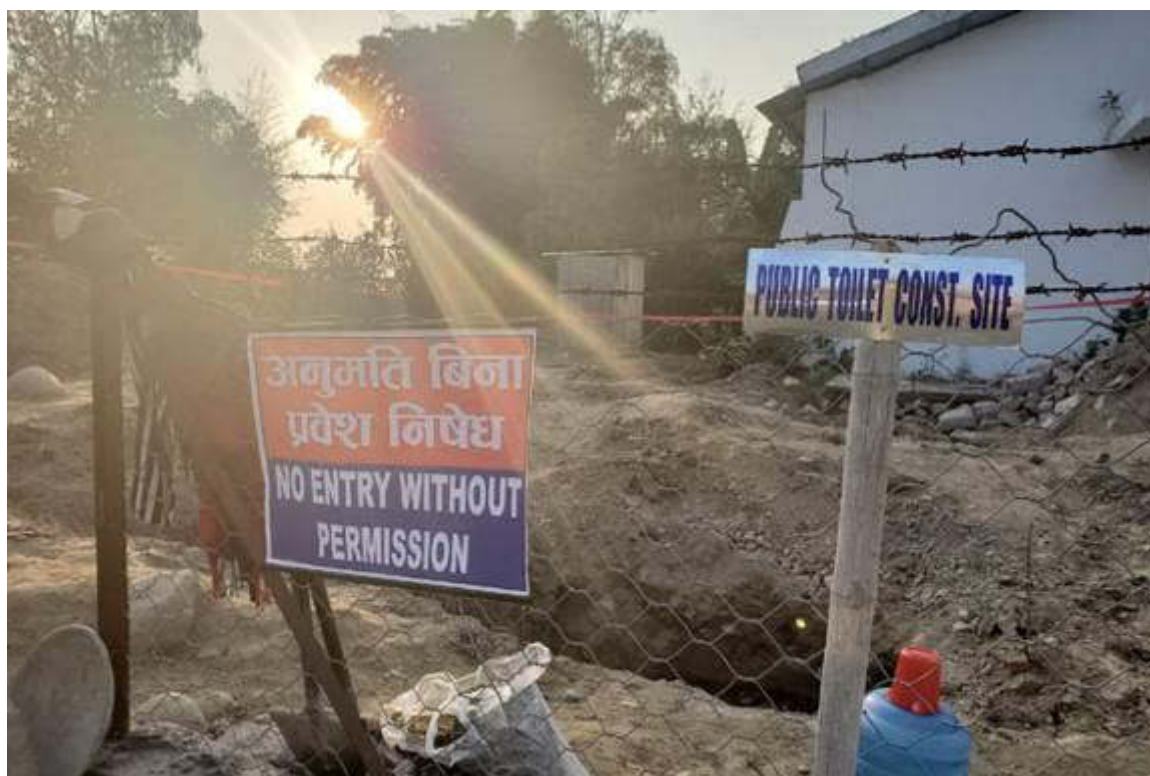
Public Toilet construction site in ward 8 of Rapti rural municipality
