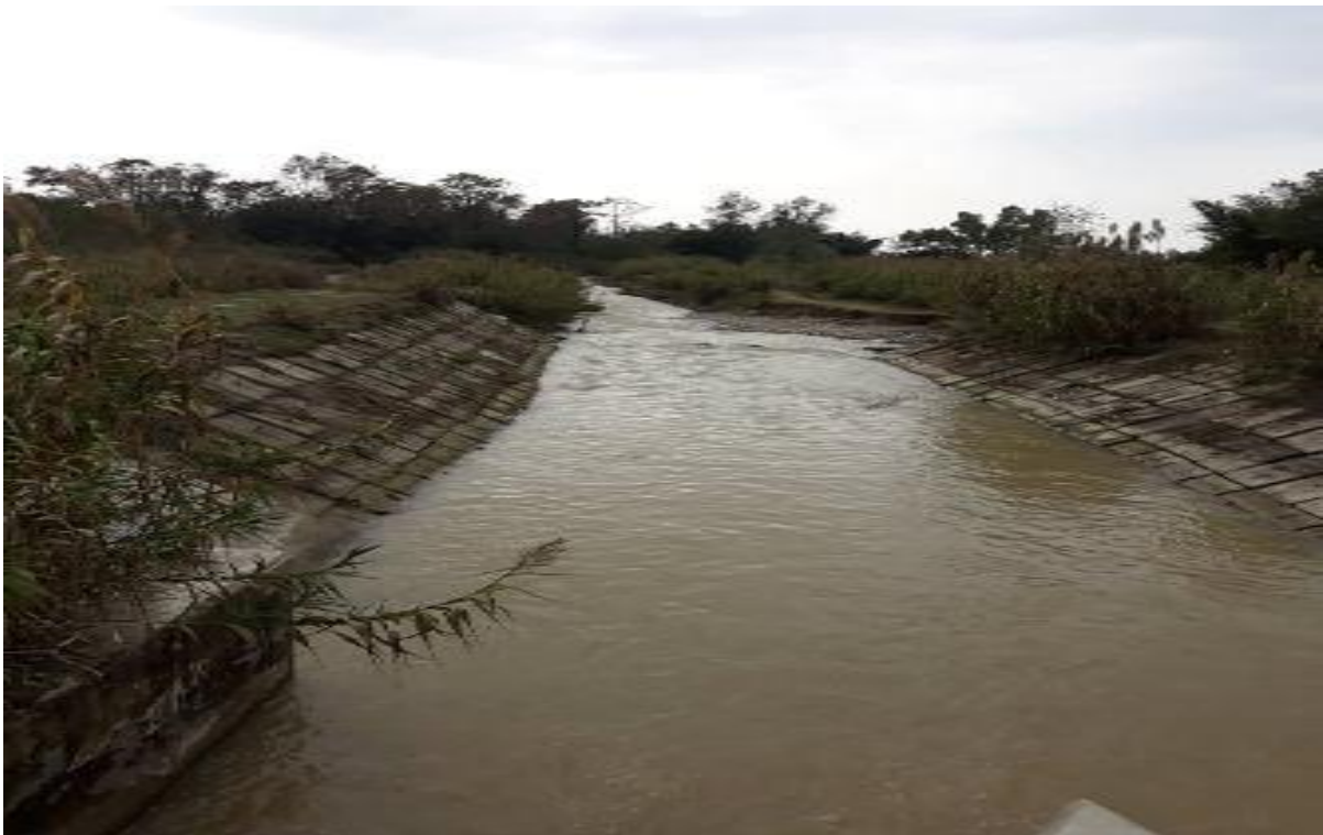
Outfall location at South Gyani Kulo of Tikapur municipality ward no.1,
