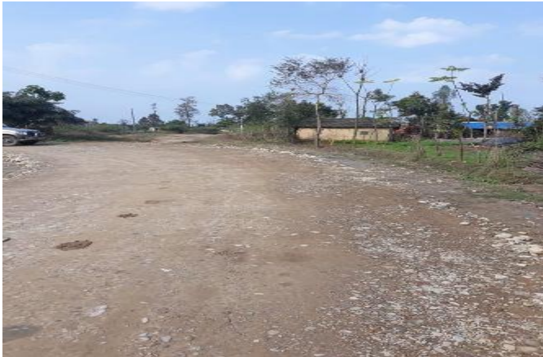
Proposed public/government Road ROW for Drain construction at Shaktinagar area, Tikapur municipality ward no.1
