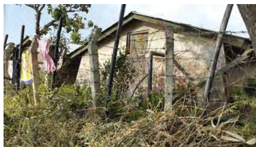
2. Existing RVT at Base Camp
