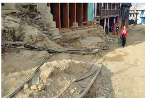
5. Existing Condition of Distribution Pipelines
