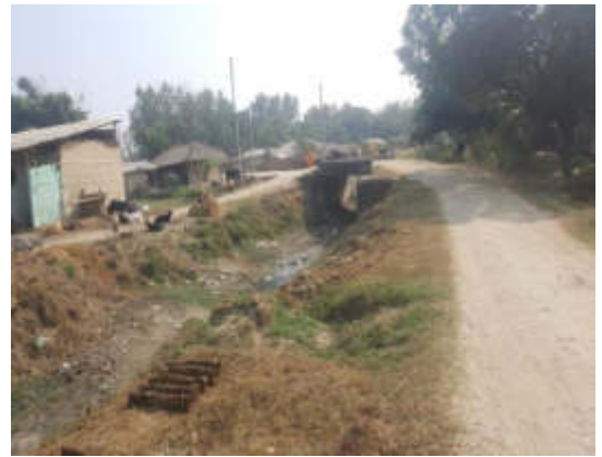
2. Outfall at Canal
