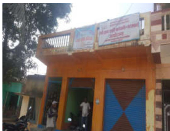
6. Project Implementation Unit Office, Rautahat
