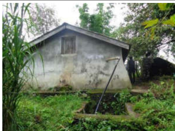
6. Existing RVT at Gadithumka
