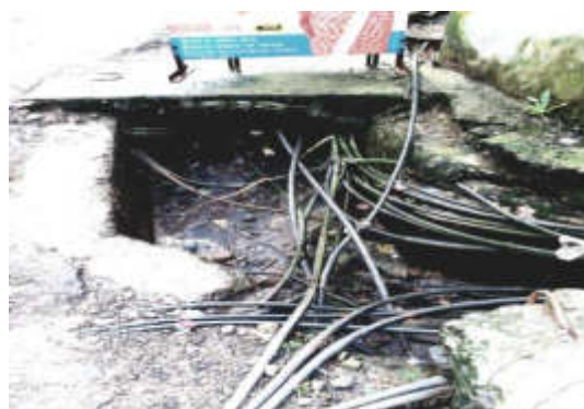
8. Existing condition of distribution pipelines
