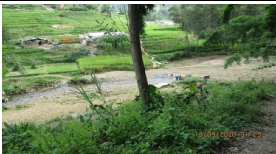
Photo 18: Proposed GRVT construction site with boring near bank of Mahadev khola, WN 4
