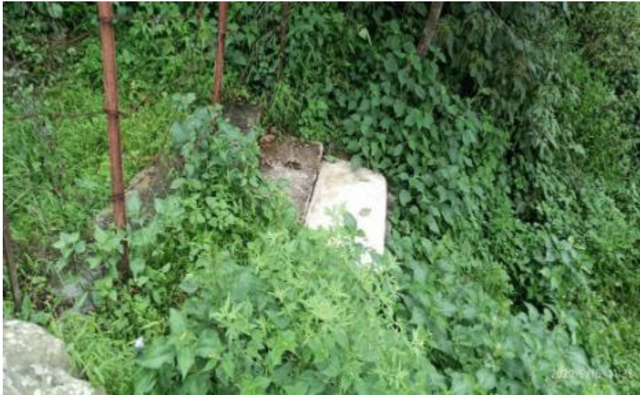
Photo 19: Proposed spring intake site at existing spring intake, Syangtang - WN 4
