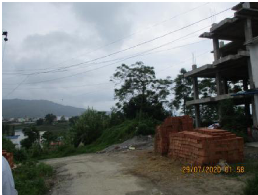
Photo 17: Proposed site for construction of 2 GRVTs, pump house, guard house, WTP at Pandhera, WN 4
