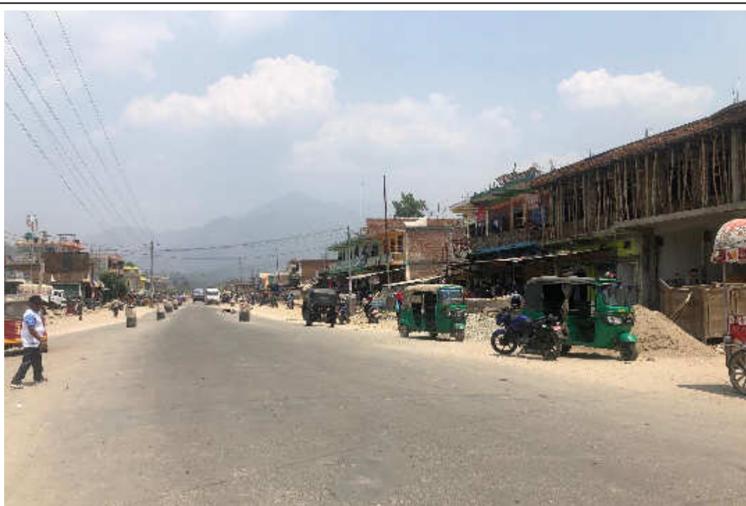
Photo 8: A project area site where water will be supplied through distribution lines
