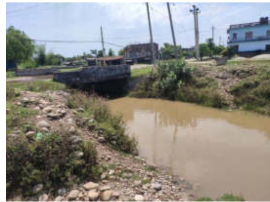
Photo 8: Outfall of Block 18
