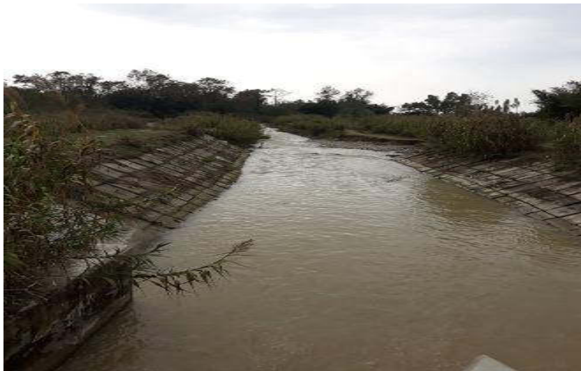
Photo 2: Outfall Location at South Gyani kulo, ward number 1
