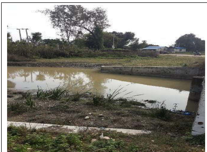
Photo 1: Outfall Location at North Gyani kulo, ward number 1
