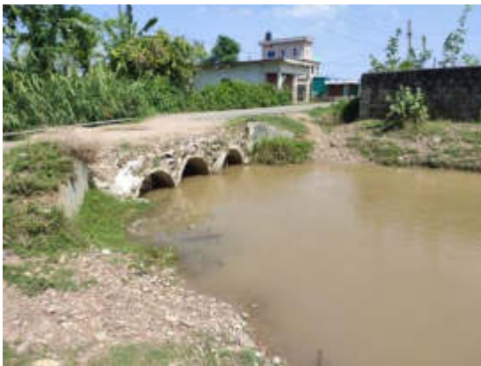
Photo 9: Outfall of Block 19
