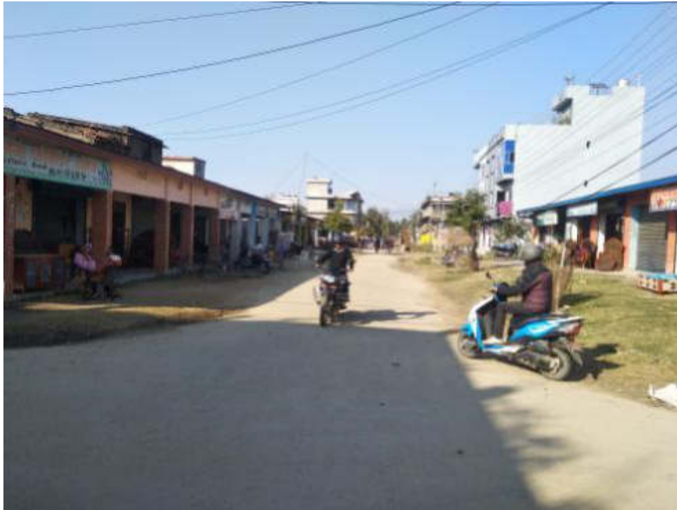
Photo 1: Storm Water Drainage service area (Park Road, Ward 1)
