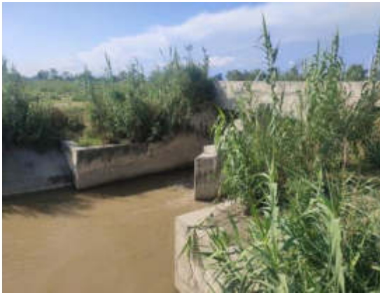
Photo 5: Main outfall of Banagaun area to Jamara Canal
