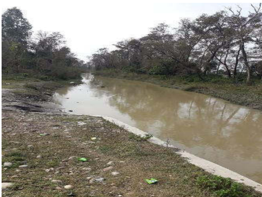
Photo 4: Outfall Location at South Gyani kulo, Shanktinagar area
