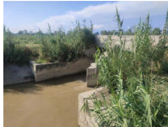
Photo 6: Outfall of Block 8
