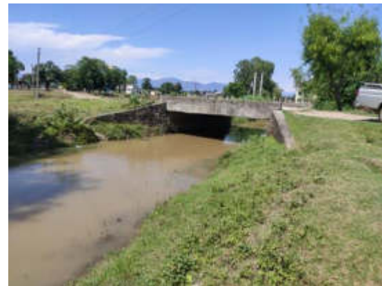
Photo 10: Outfall of Block 21
