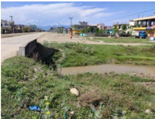
Photo 7: Outfall of Block 12
