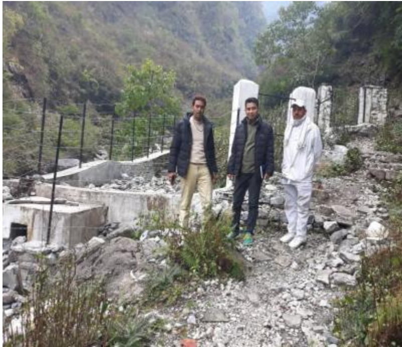
Photo 3: Existing Intake site of Khalanda sub-system
