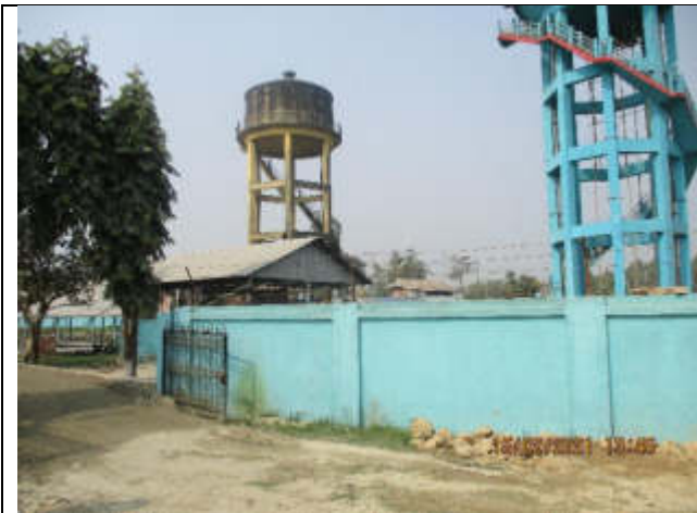
Photo no. 1: Existing OHT,(100 Cum) in WUSC compound at Pani tankey Ramdhuni Municipality ward no 3
