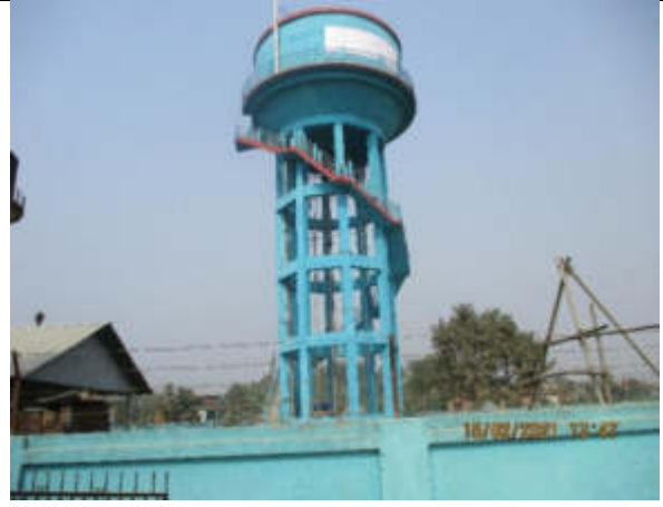
Photo 2: Existing OHT, (225 Cum) in WUSC compound at Pani tankey Ramdhuni Municipality ward no 3.
