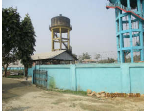
Photo 1: Existing OHT,(100 Cum) in WUSC compound at Pani tankey Ramdhuni Municipality ward no 3.
