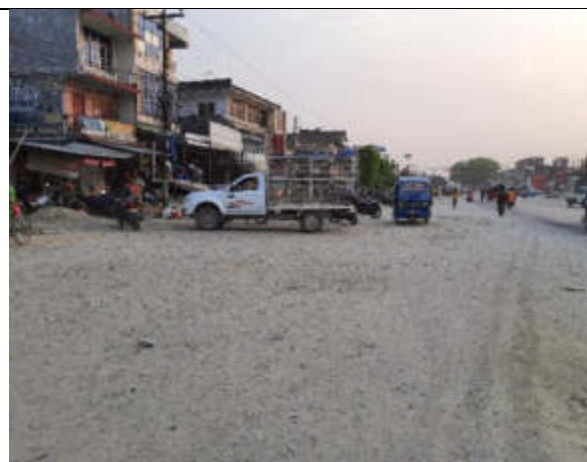
Photo 18: Road along which Pipe line traversed for the main and distribution networks
