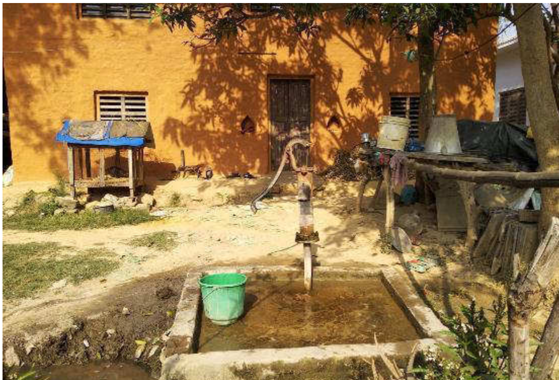
Photo 6: Existing shallow tubewell in project area
