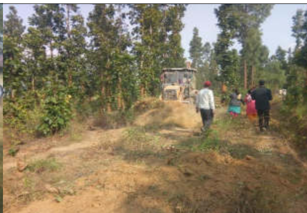
Photo No.6: Observation of access road construction site, Shubhaghat, Surkhet
