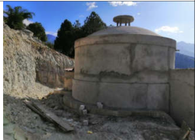
Photo No.3: Constructed RVT, Bajhang
