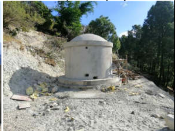
Photo No.4: Constructed Collection Chamber, Bajhang
