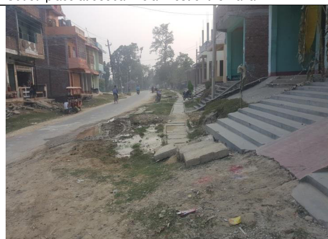
Service area Shajha chowk , with existing drainage
